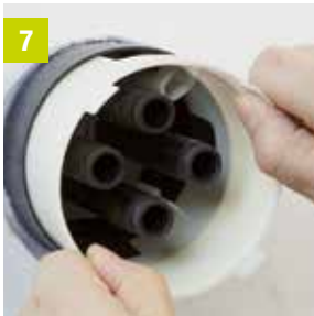
Remove assembly pipe
